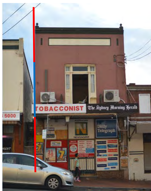
Figure 27: Measurement of 3.447 metres from ground level to the underside of the awning (represented by each alternating red/blue line)
