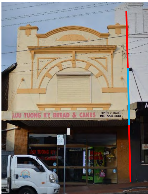
Figure 24: Measurement of 3.096 metres from ground level to the underside of the awning (represented by each alternating red/blue line)
